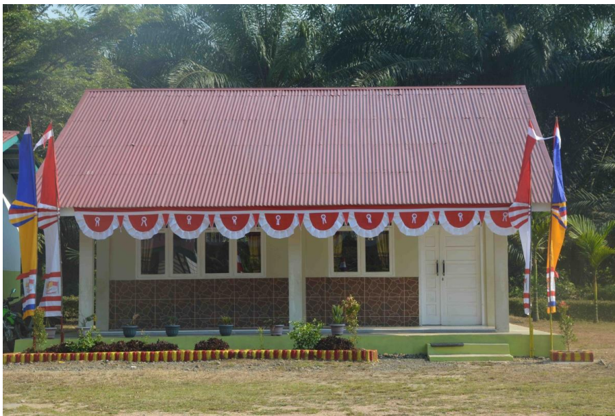
Front facade of the library building of SD Swasta YTKA 03, Gunung Tujuh, Desa Kemarau.
